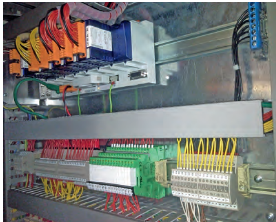
▲ Installation of new PCD's in an existing cabinet
