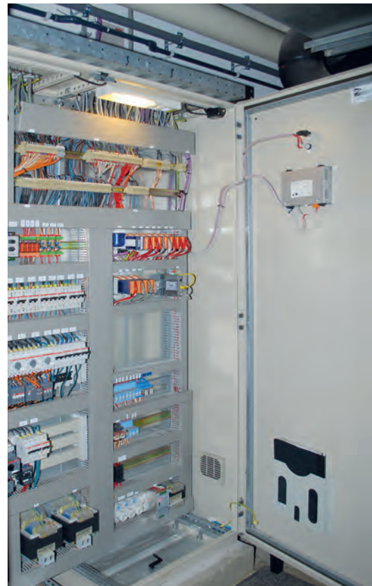
▲ Enough space left in cabinet by the old controller
