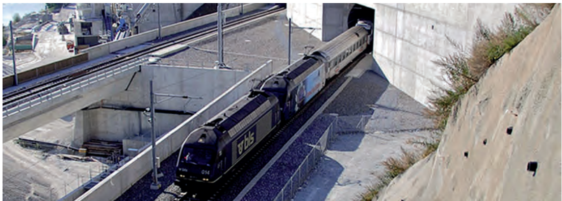
▲ Two single track tubes connected by cross tubes all 333m South portal near Visp (Wallis)
