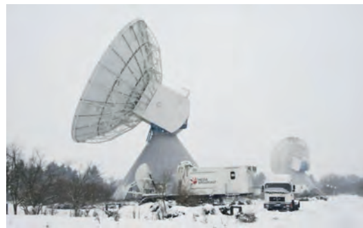
◀ Intelligent antenna heating
