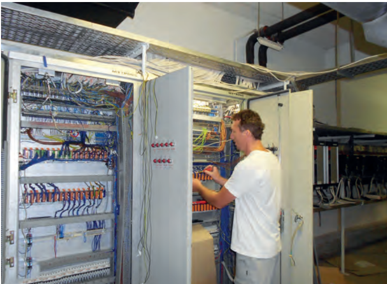
◀ The new system during setting
