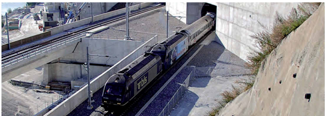
▲ Two single track tubes connected by cross tubes all 333m South portal near Visp (Wallis)
