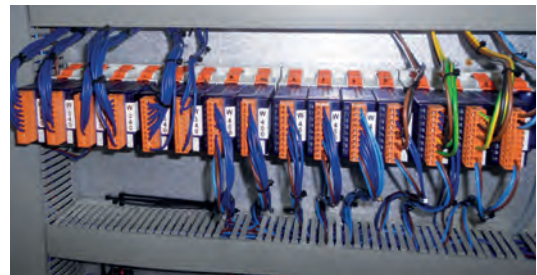
▲ The new system during setting
