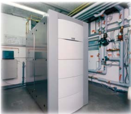
Photo: Vaillant GmbH fuel cell heater in a field test under normal working conditions
