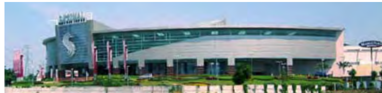
«Lindeteves Mall» shopping centre in Indonesia
