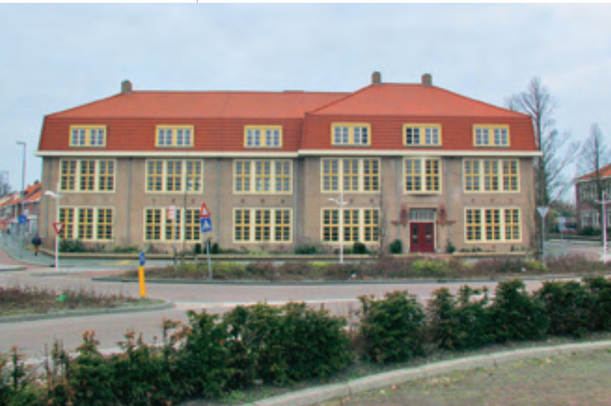
Outside view of the renovated company headquarters of "Woningstichting Den Helder"
