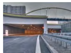
City tunnel in Poland 72
