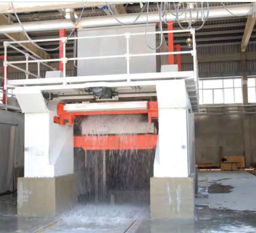
The tough industrial requirements of the marble industry
