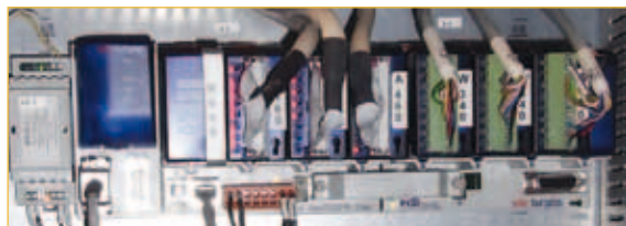
Saia®PCD3 with SD flash card module Saia®PCD3.R600 in the post and freight terminal
