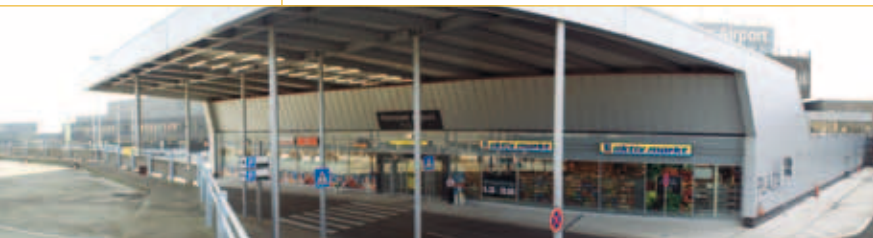
Airport Plaza parking deck
