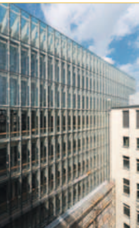
The large window frontage allows optimum use to be made of daylight
