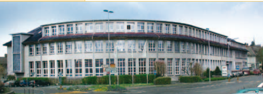
Saia-Burgess Controls Headquarters at Bahnhofstrasse 18 in Murten (Switzerland)
