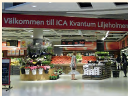
Four sophisticated refrigerators are monitored with SaiaVisi.Plus in a supermarket in Sweden.
