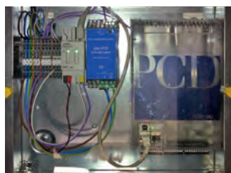
▶ PCD1.M2120 EIB/web connection to the existing EIB network
