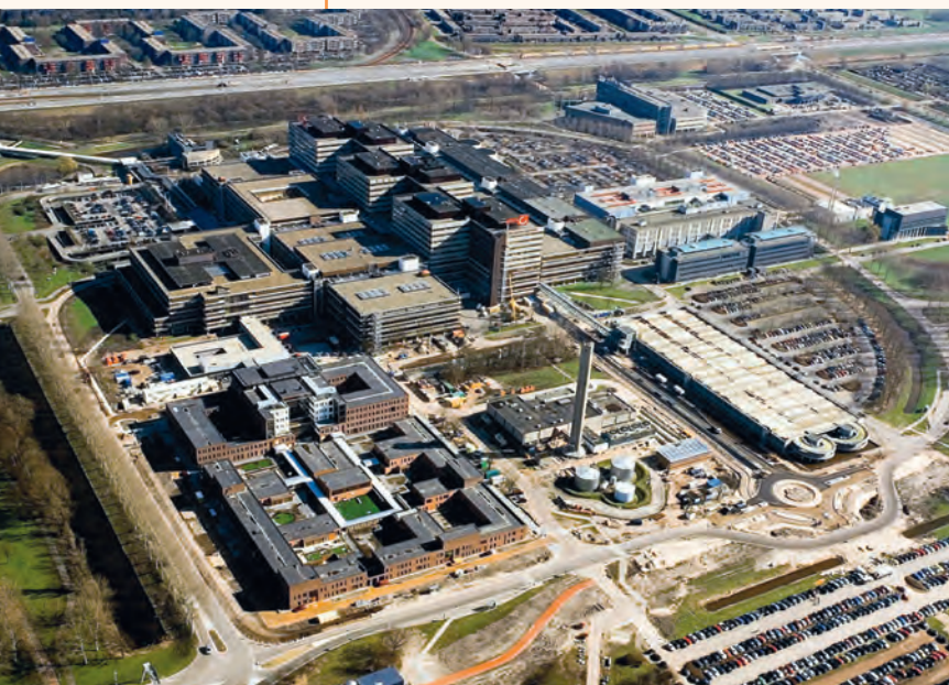
▲ Aerial view: AMC Hospital Amsterdam
