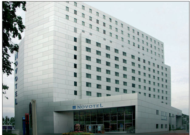
Novotel, Bern | BEA Expo Knowledge of the user's energy requirement is important for energy management in hotels, motels, hostels, hospitals, etc.
