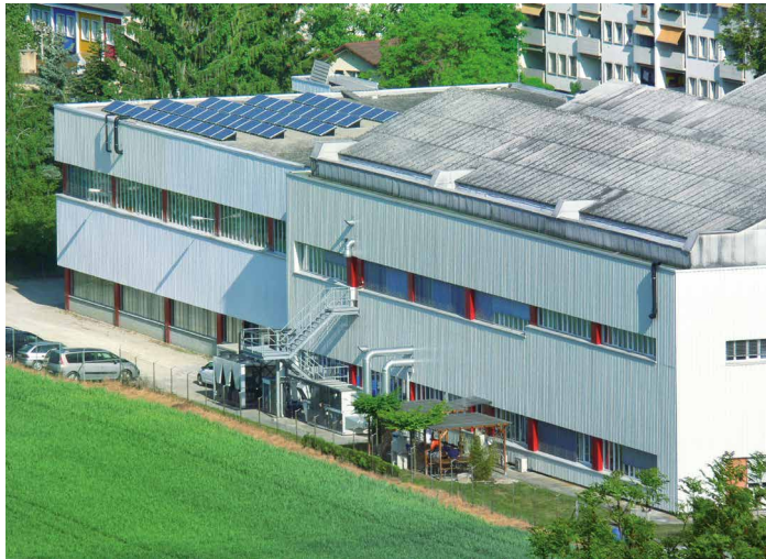
Factory 2: SMD Production and Small Devices Business Area. Solar plant with 11 kWp for "green" air conditioning
