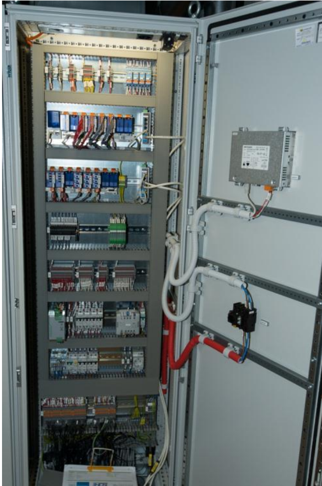
Control cabinet with PCD3.M6860 and 5.7" Micro-Browser Panel
