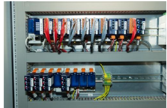
PCD3.M6860 with 2 x Ethernet, BACnet PCD7.R561, PCD3.R600 SD-Flash, Manual override I/O modules
