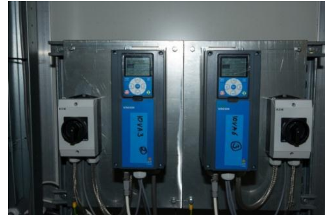
Frequency converter with Ethernet Modbus-TCP interface
